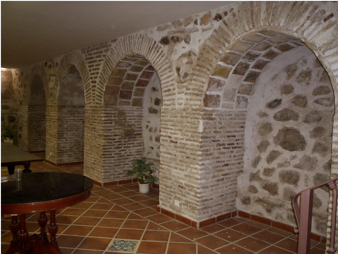
Fig. 10. Arches of the underground gallery closed by a support wall. Photograph by Victoria Soto Caba.
