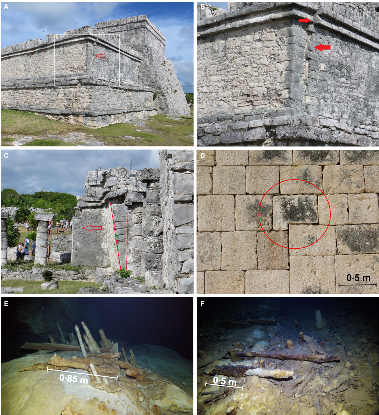
Fig. 11. Evidence of palaeoseismicity in the Yucatán Peninsula. (A) to (C) Correspond to archaeoseismological features described by Rodríguez-Pascua et al. (2011) as primary effects that occur when the ground transmits seismic waves to buildings. (A) and (B) Displaced walls at the Tulum archaeological site (main building height 12 m). (C) Tilted walls in a structure at the Tulum archaeological site (column height 1.90 m); tilting occurs as a consequence of horizontal ground movement which affects the wall foundations. (D) Reconstruction techniques as the result of previous seismic activity producing intense ground shaking. This reconstruction is observed at Chichen Itza archaeological site. In this case it consists of interlocked blocks, usually used as a reconstruction technique after seismic damage, as has been observed in other areas of Mexico (Giner-Robles et al. , 2012). (E) and (F) Effects of palaeoseismicity present in submerged cave systems from Quintana Roo. (E) Tilted, collapses and orientated speleothems in the Tajma Ha cenote. (F) Collapses and orientated speleothems in the Minotauro cenote.
