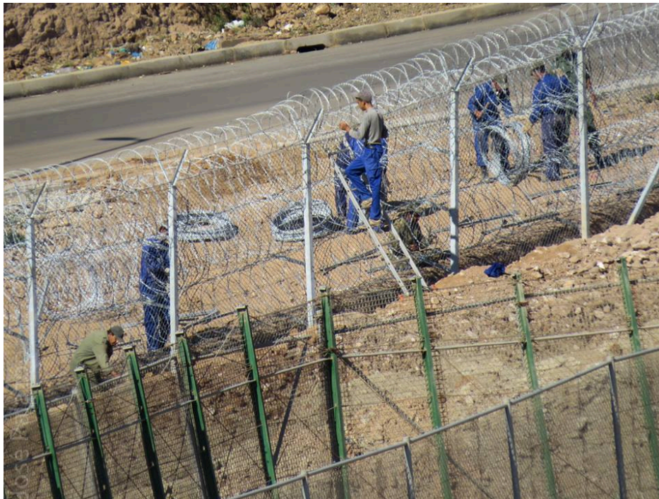
Figure 4.8. The construction of the fence on Morocco's side (Melilla)
